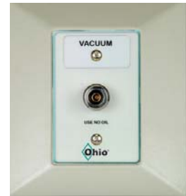
DISS Wall Outlet DISS Ceiling Outlet
